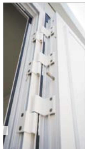
detail hinge system with locking doors
