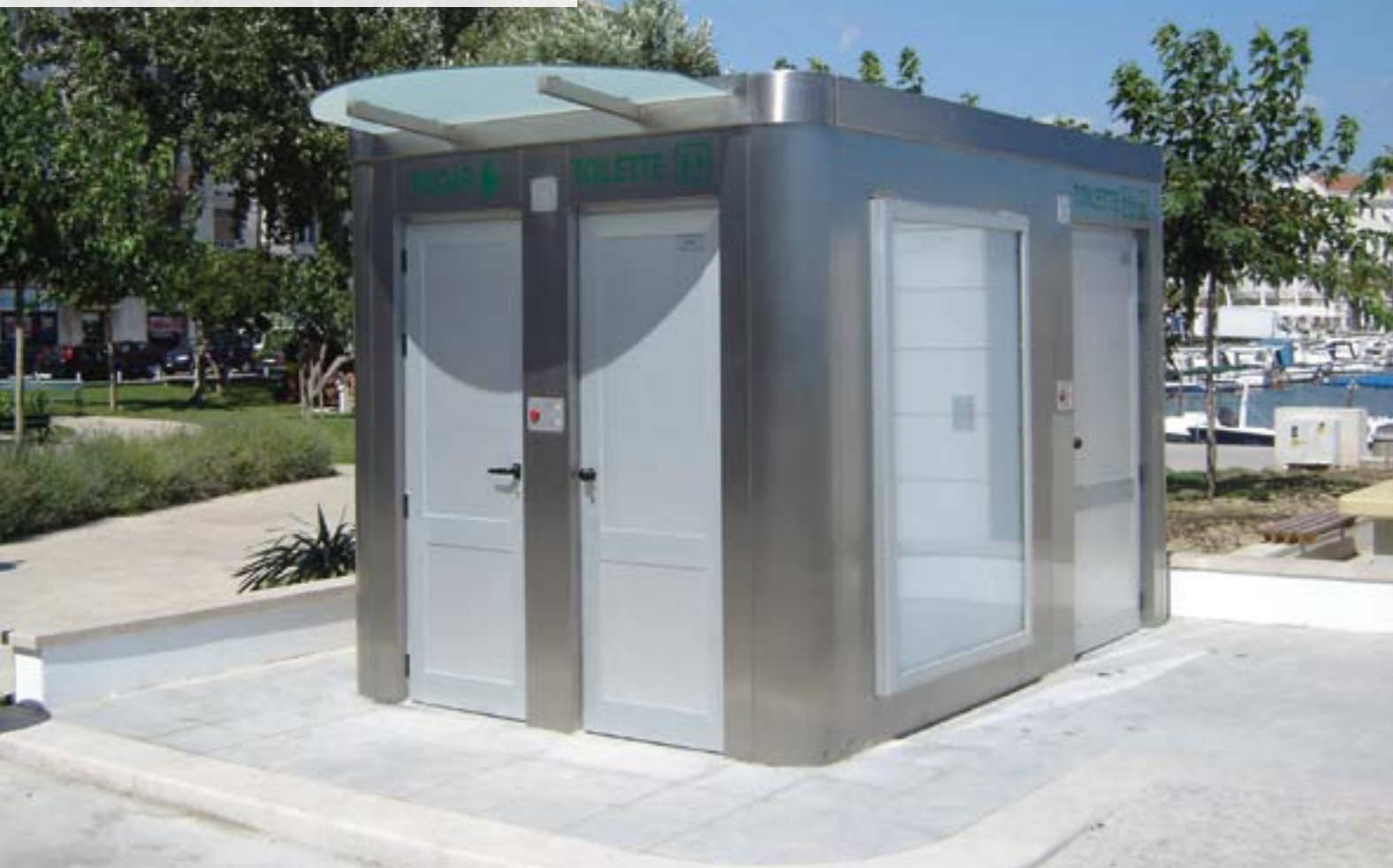
Classic toilet with three user-space (people with disabilities, men, women) with gray facade similar to stainless steel, Röttenbach, Germany
