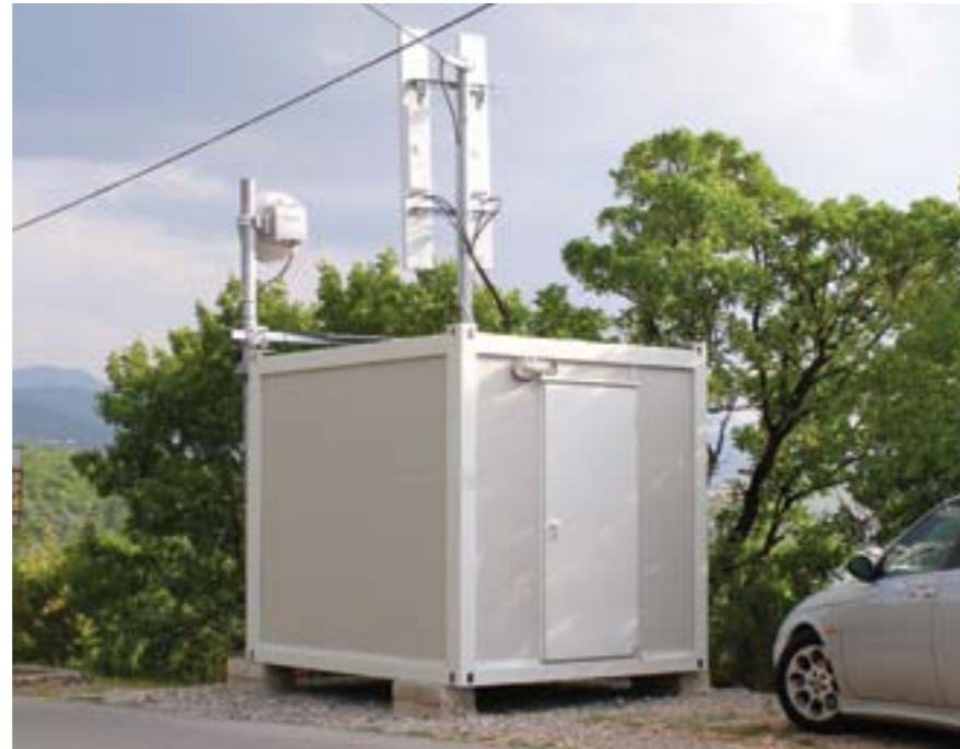
container for electronic and telecommunication equipment (fixed and mobile - GSM), television signals, air traffic, railway or roadtraffic, or air pollution control unit
