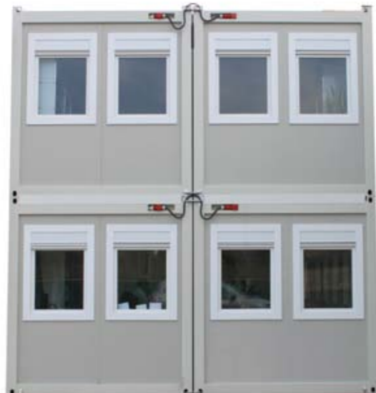
Group system of modular construction container facility on location
