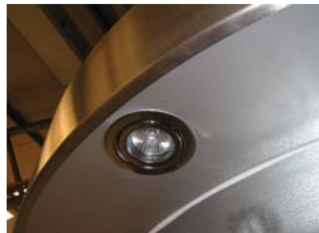
halogen illumination in stainless steel roof
